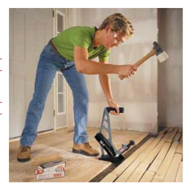
Sequential Actuation Trigger (also known as restrictive trigger or trigger fire) operates in the following a sequence - depress the safety element at the nose of tool against the work surface then pull the trigger. After each fastener is driven, release the trigger and lift the tool off the work surface before starting the sequence again. This trigger is recommended and acceptable for most applications.
